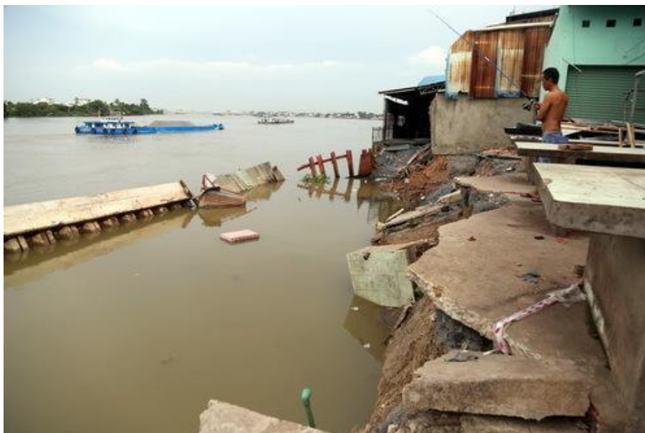
Figure 3-30 Broken dike along Dong Nai River bank
